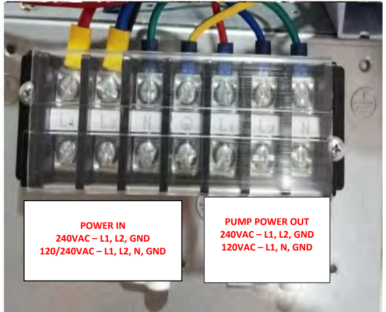
Connect Main & Pump Power
